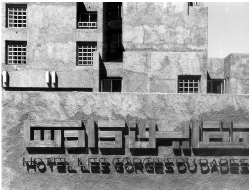
Wooden sign made by Mohamed Chabâa, Hotel Les Gorges du Dades, Boumalne, 1970-71. Architects: Faraoui et de Mazières, © Cabinet Faraoui et de Mazières.
