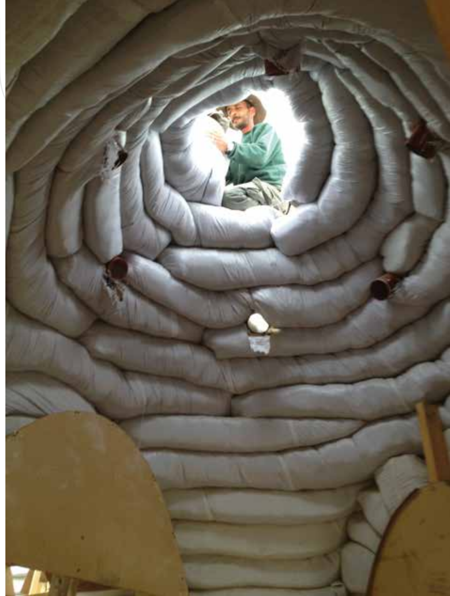
Finishing the dome.
