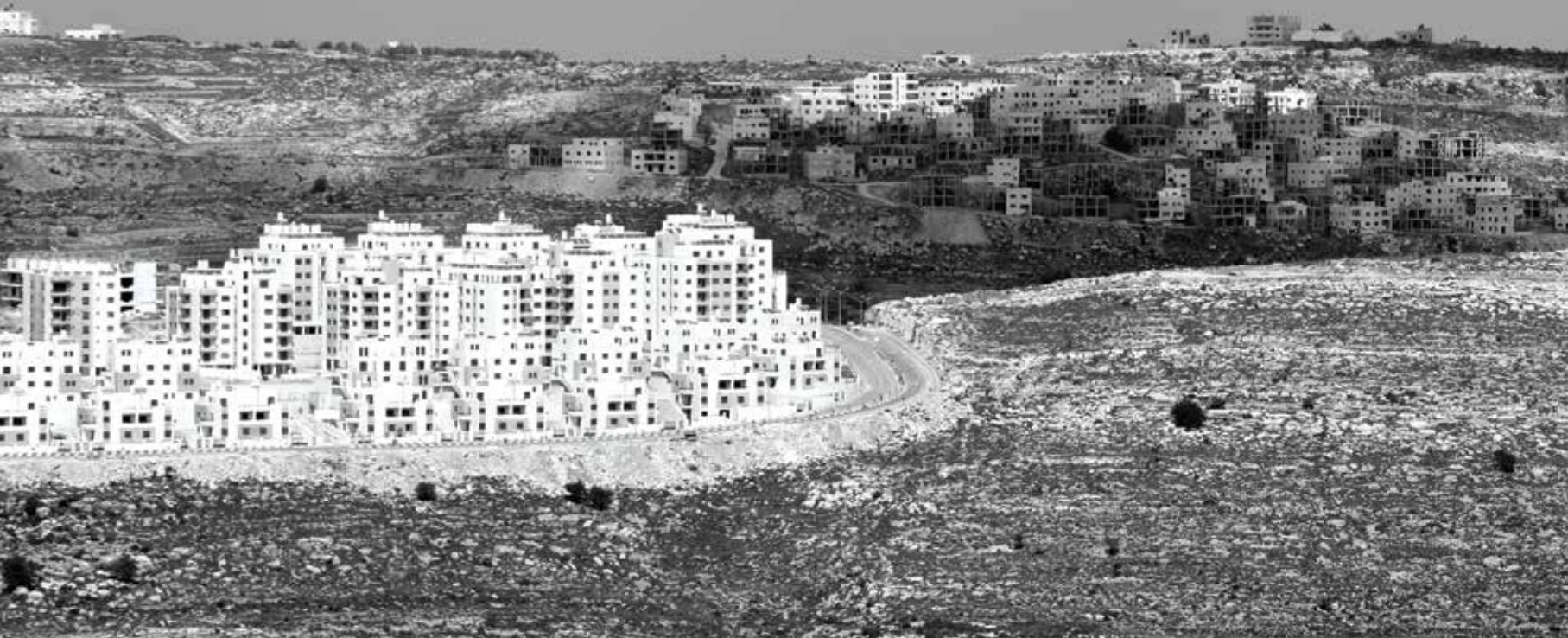
Al-Reehan Neighborhood, in its shadows rise skeletons of an abandoned mid-90s development site.
